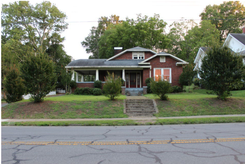
Front Slope of Union Street Wall Location
